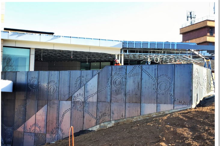
Installation of the Coreten steel entrance walkway piece.
