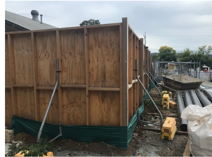
Photo 6 – Hoarding that act as noise barrier was installed along the perimeter of the Community Hall.
