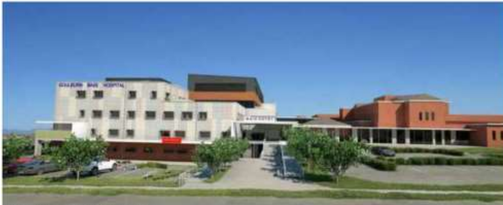
North View, Previous Scheme
