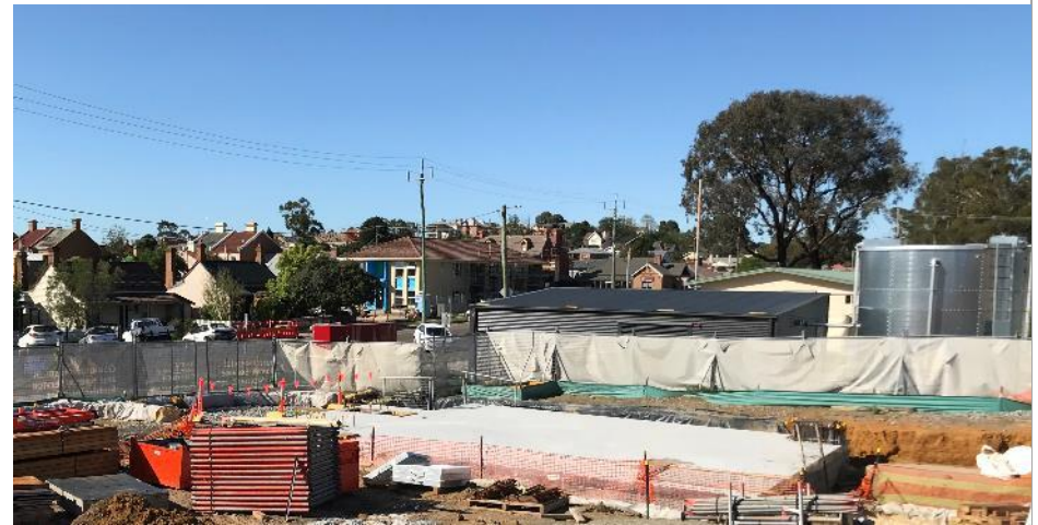
Photo 6 – Erosion and sedimentation controls at the low point area of the site
