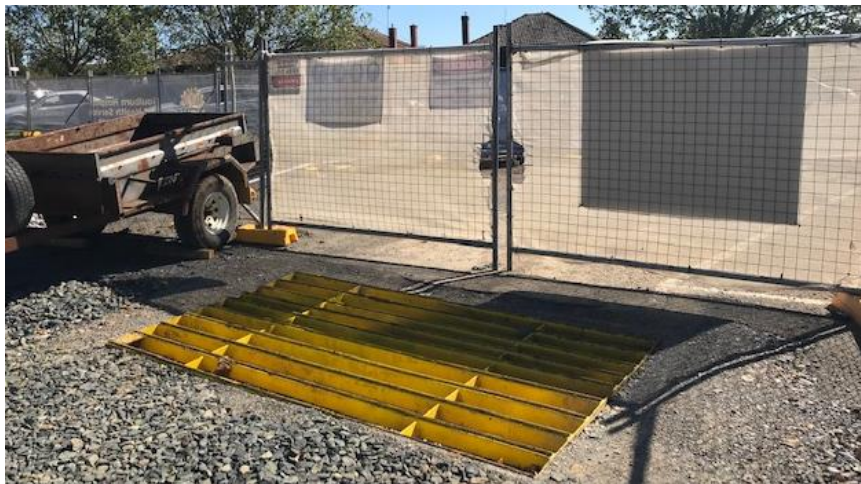
Photo 3 – Rumble grid in place at the site entrance
