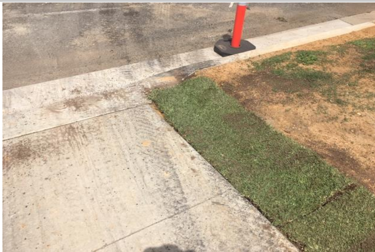
Photo 7 – Footpath batter at site entrance has been turfed and seeded.
