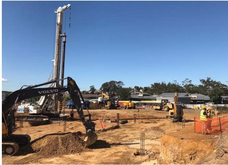
Photo 9 – Current works onsite – piling works and drainage works.
