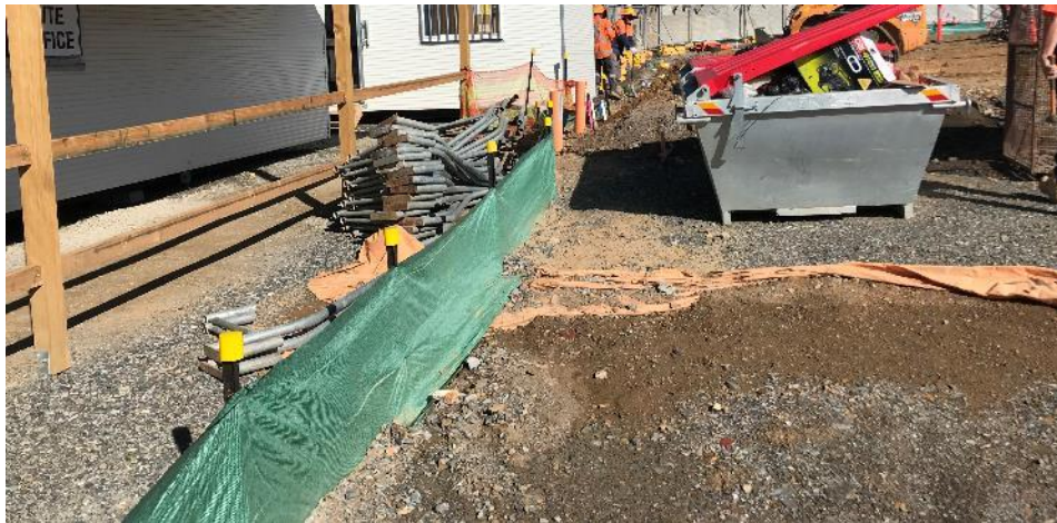
Photo 5 – Sediment fencing was installed around the perimeter
