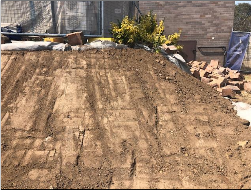
Photograph Post excavation and geotextile barrier evident on battered walls note varying depth of excavation to accommodate future site works
