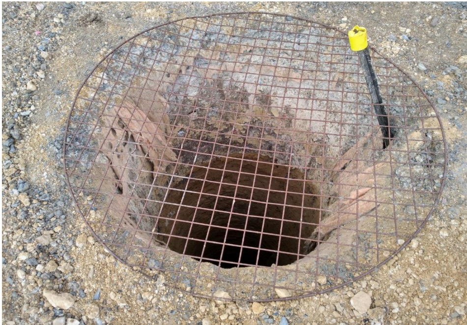
Photograph □□Typical piling hole□
