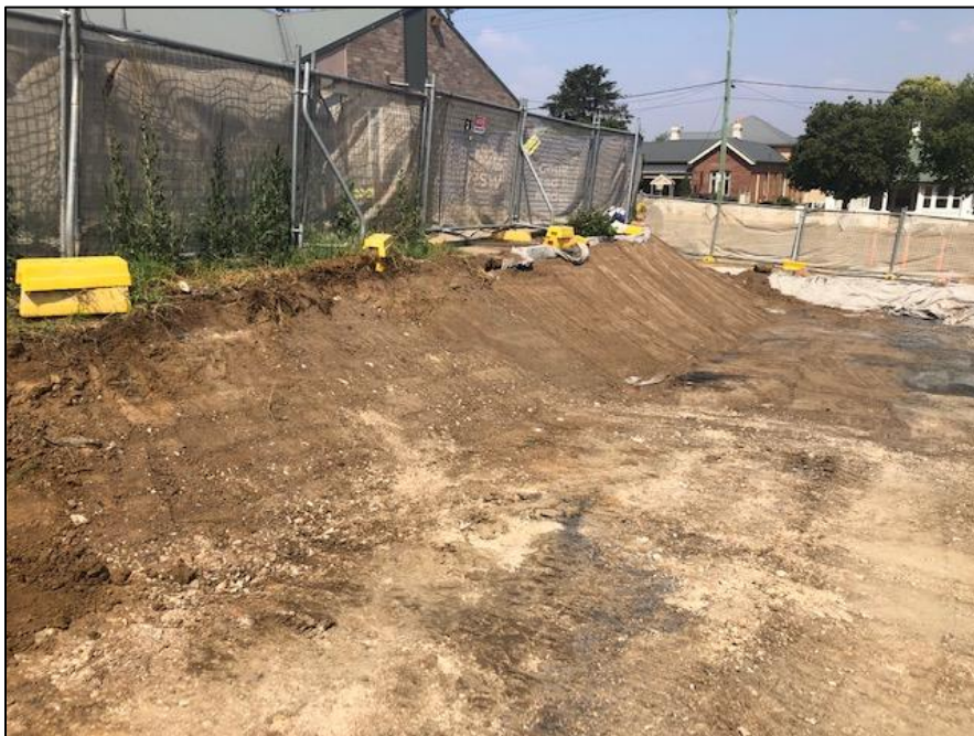
Photograph Post additional excavation and battering
