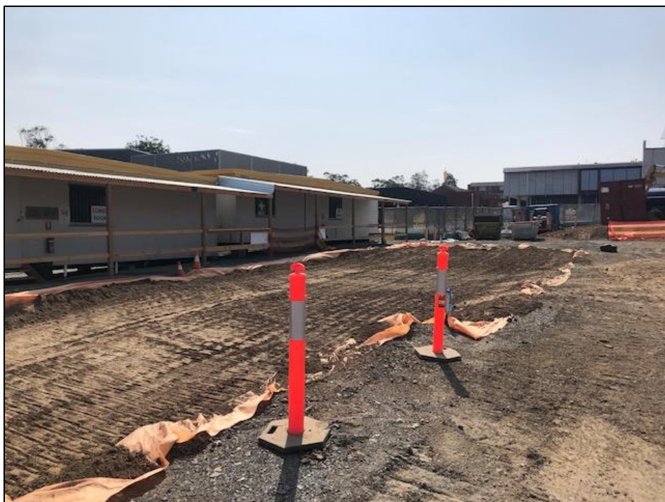
Photograph 2 Post excavation and geotextile liner evident and use of clean fill.
