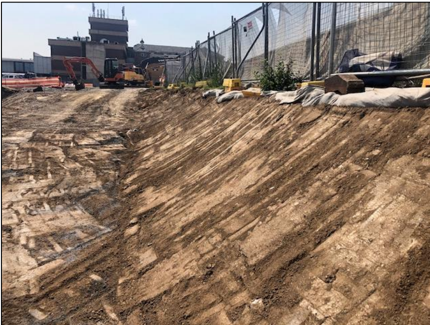
Photograph Post excavation and geotextile barrier evident and use of clean fill
