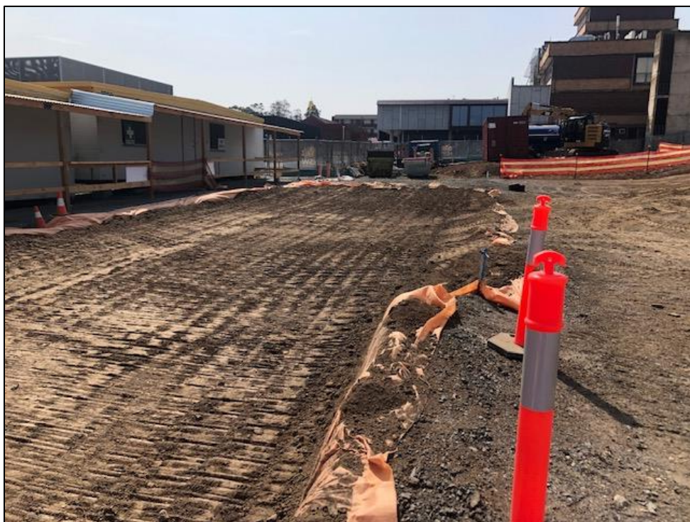
Photograph Post excavation and geotextile barrier evident on pit walls.
