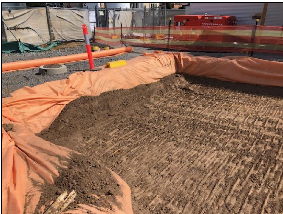
Photograph 1 Post excavation and geotextile liner evident on pit walls. Not varying depth of excavation to accommodate future site works.
