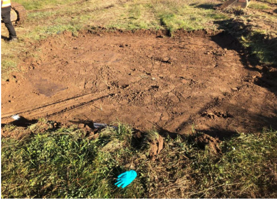
Photograph 1: Final excavation at Test Pit 8 (looking west).
