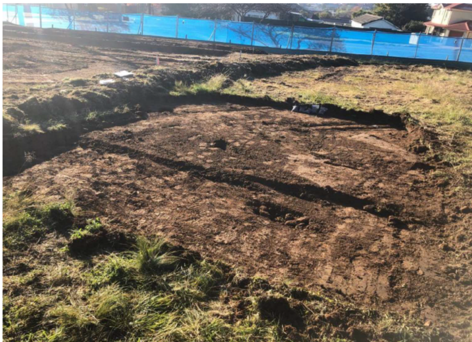
Photograph 2: Final excavation at Test Pit 8 (looking east).
